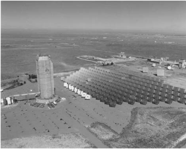
Fig. 1. National Solar Thermal Test Facility at Sandia National Laboratories in Albuquerque, NM. The heliostat field covers an area of about 160 m by 260 m.
